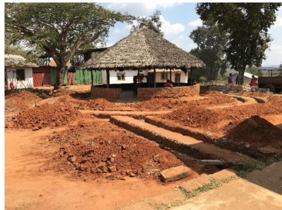
The “banda” and new paths under construction at the Orphanage
